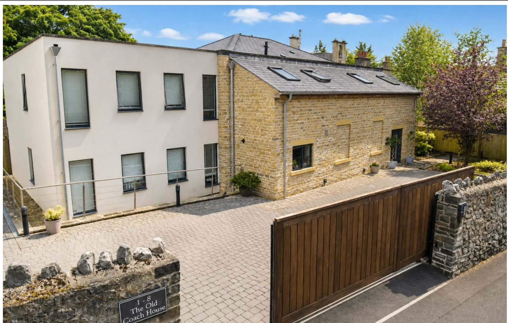
APARTMENT 1, THE OLD COACH HOUSE HOLMWOOD WESTBURY ON TRYM BS9 3FG
